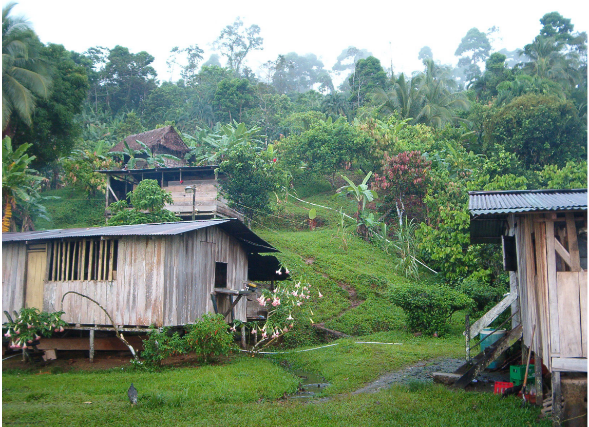
Figure 8: Photo of standard style houses in the Cayo Paloma area.
