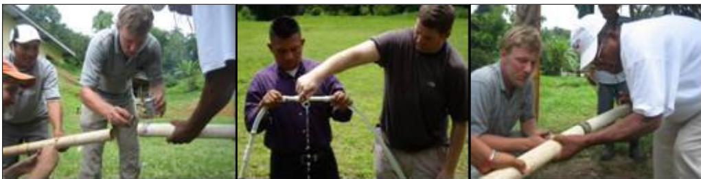
Figure 3.2 – Session two focused on skills such as gluing PVC joints and learning ways to remove air and debris from tubes. Source: Photos by author
