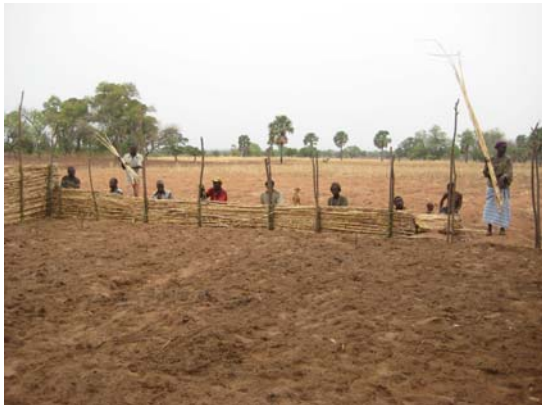
Figure 9: (left) Building the Fence (photo provided by Olga Y. Castro)
