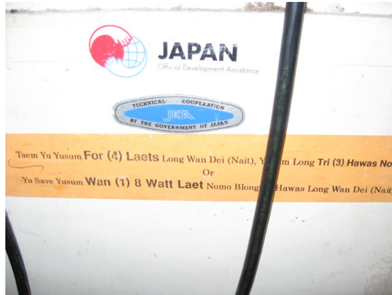
Figure 4.4: Lights usage guidelines placed near the charge controller and battery.
