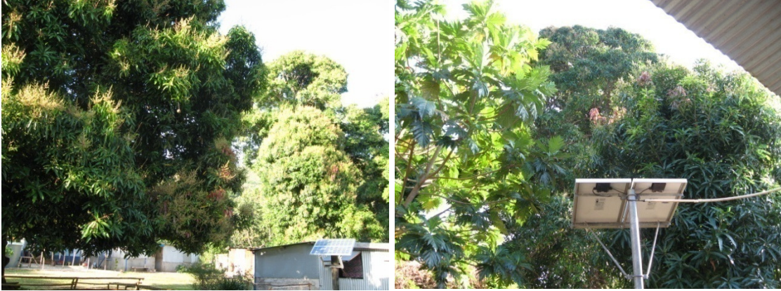
Figure 4.1: Examples of shading of solar panel
