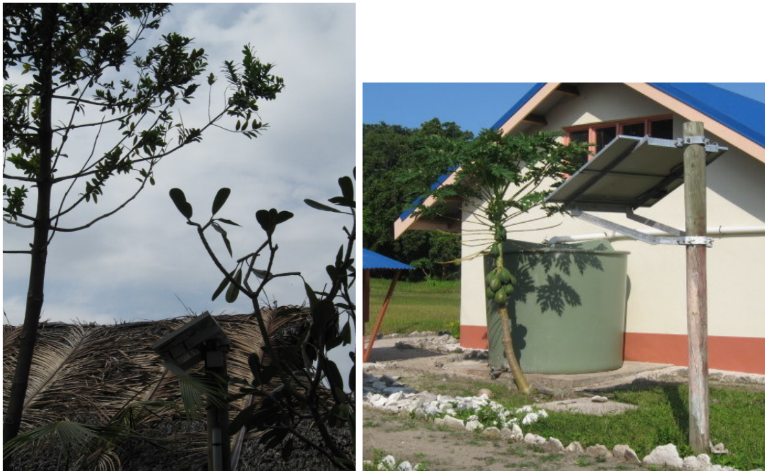
Figure 4.3: Tree saplings near solar panel location in the beginning of installation resulting in almost total shading after a few years. Author advised cutting down the offending trees in both photos and neither were cut down.
