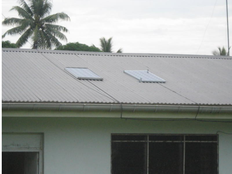
Figure 4.2: Example of community institution self-install. Panels are facing the wrong direction and mounting directly on tin roof results in overheating the panels, significantly reducing power output.
