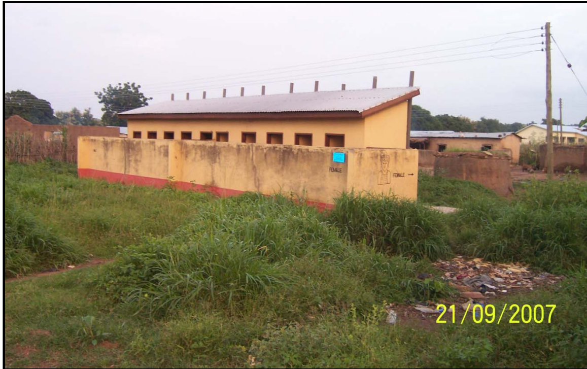
Figure 5: Photograph of an institutional latrine in Ghana
