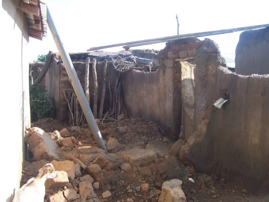
Figure 53: A collapsed superstructure, in this case the vent pipe remained intact
