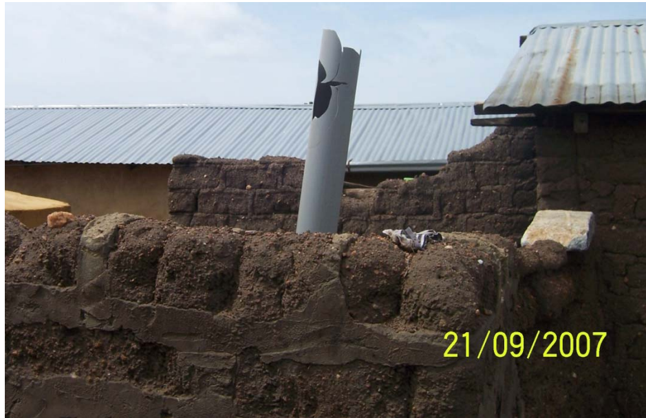
Figure 54: A broken PVC vent pipe, cause unknown
