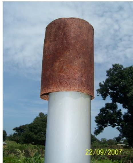
Figure 56: A capped vent pipe
