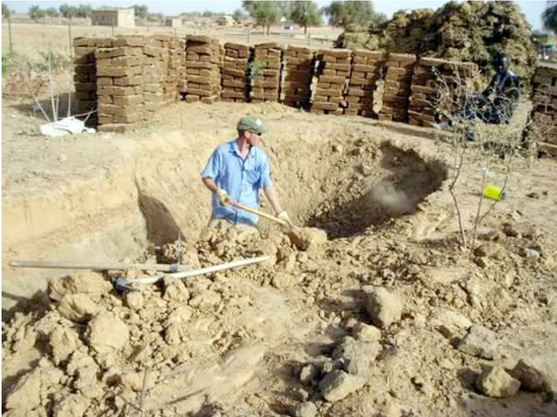
Figure 20: Digging the first fish pond
