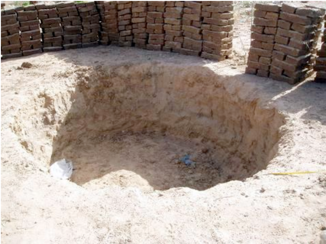
Figure 19: Initial hole for the fish pond
