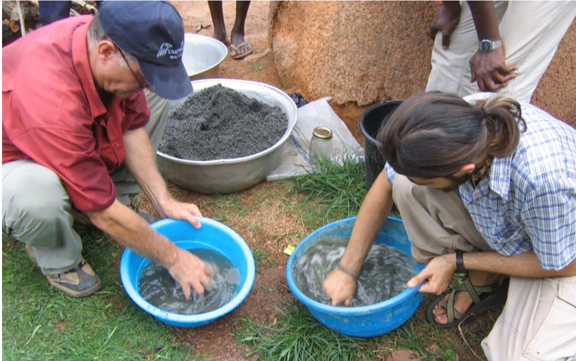
Figure 23: Washing of the filter media in small batches
