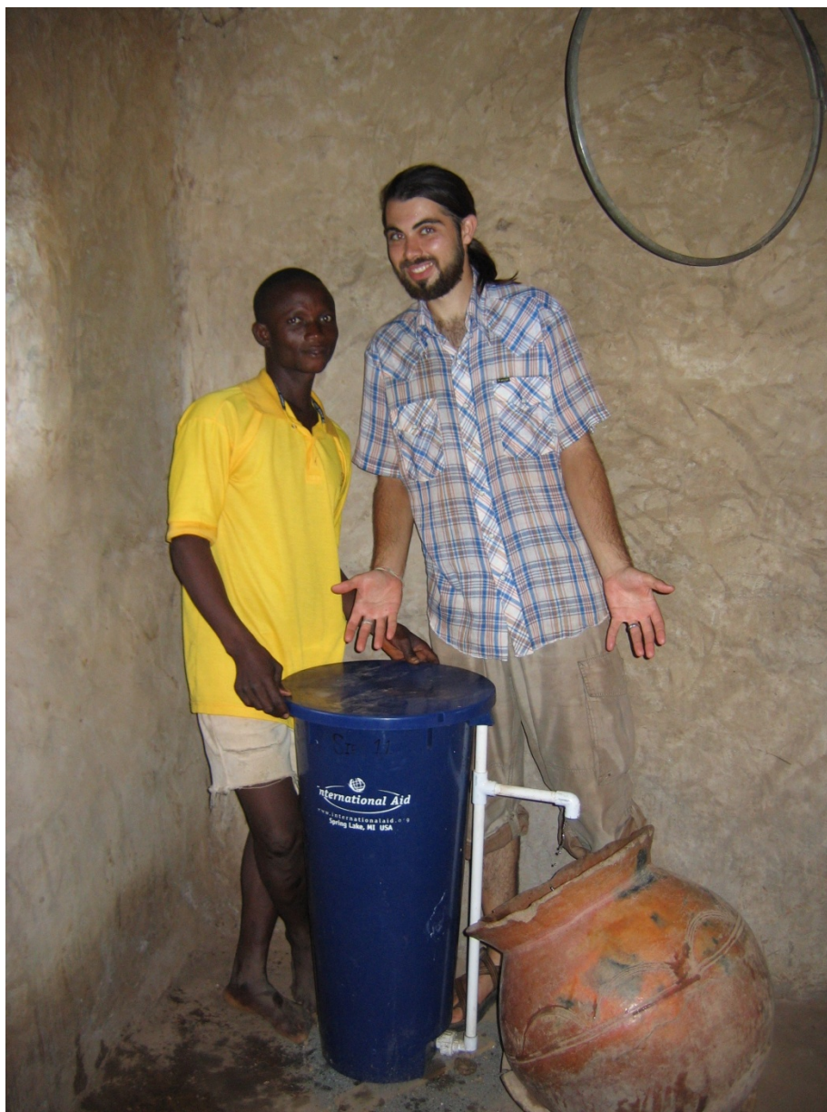
Figure 36: BioSand Filter owner Stepen Agba chose to install Sibi 11 in an alcove of his house to be protected from the weather, and collect his water in a ceramic pot to keep the drinking water cool
