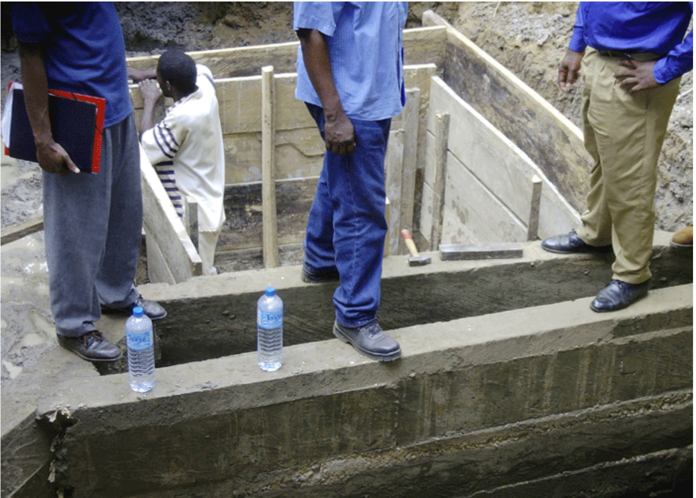
Figure 9. Construction of the Primary Filtration and Capture Area, Filter, and Reservoir.
