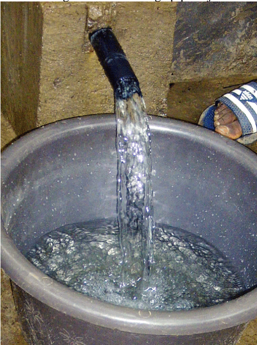
Figure 12. The Collection Pipe.
