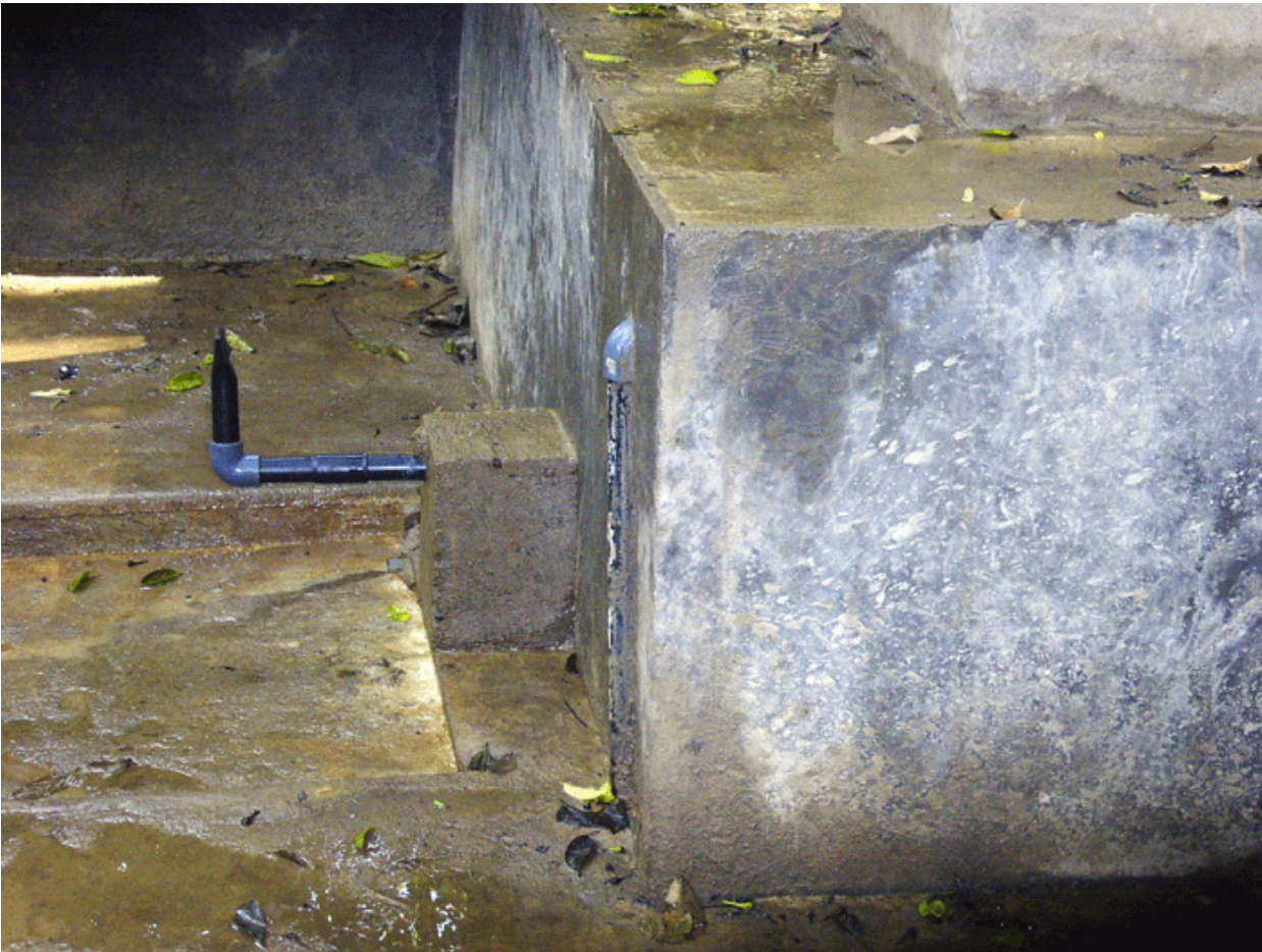
Figure 11. Reservoir with Collection, Overflow, and Drainage Pipe.
