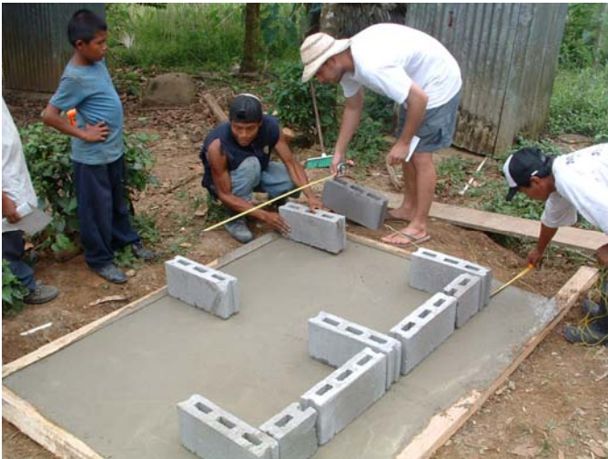
Figure 16 – Aligning concrete blocks before placing with mortar.
