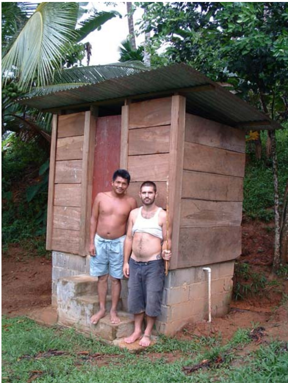
Figure 9. Typical compost latrine in the Bocas del Toro area of Panama. Note – PVC tubes (emerging from wall) transport urine from the seat to a soak pit next to latrine.
