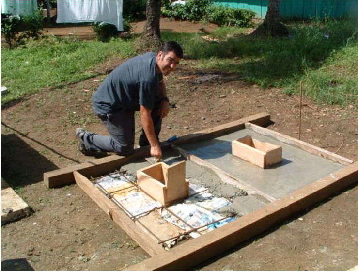
Figure 18. Construction of top floors of latrine showing wood forms to make seat holes *NOTE – Pieces or rebar, protruding upwards, can be placed in the floors at the corners to facilitate the construction of the housing structure later on (See Section 4.12).
