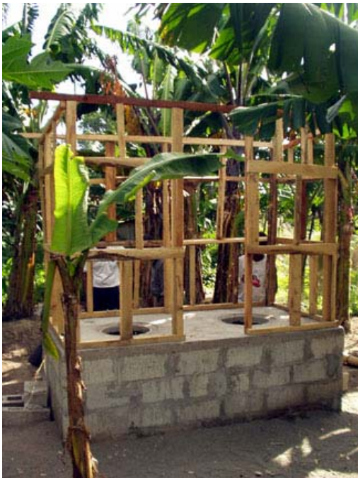
Figure 21 – Housing structure built over latrine chambers in Vanuatu, South Pacific. Concrete nails were used to connect the bottom wood beams to concrete floor. Source: Eric Tawney, PCV / Vanuatu and Master's International student
