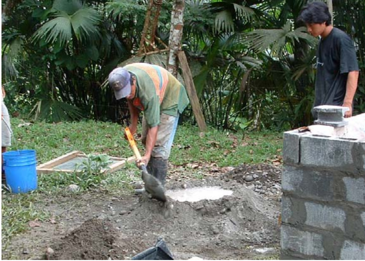
Figure 12. The “volcano” style of mixing of concrete
