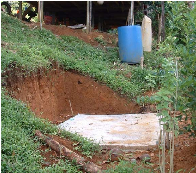
Figure 13. Leveled hillside with concrete floor of latrine showing
