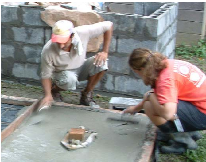
Figure 15. Smoothing out concrete with flat mason's trowel Note that people in photo are working on the top floors, but the technique is the same for the all concrete slabs.
