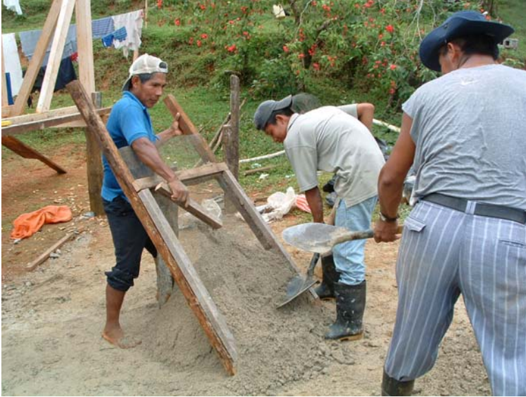
Figure 11. Sifting sand to use for mortar.
