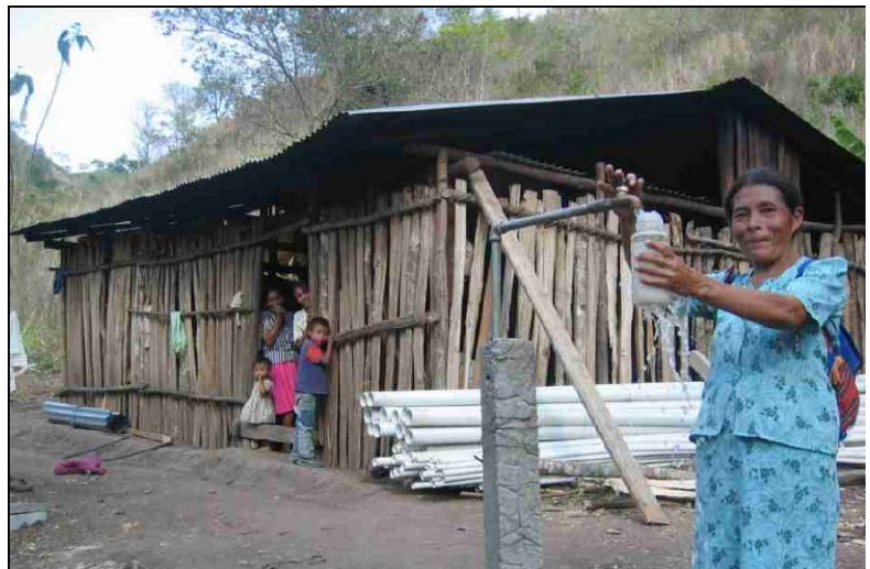
Photo 10: Water taps are installed for every home in the six communities
