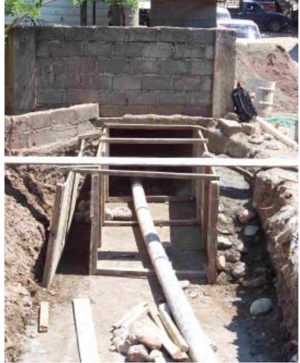
Photo 4: Formwork in question by the community where the new construction will meet the existing culvert.
