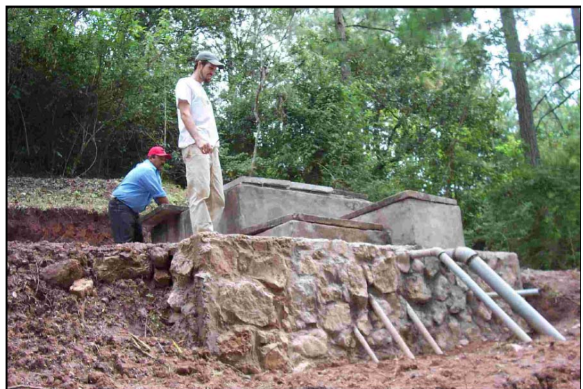
Photo 8: Rehabilitated distribution chamber
