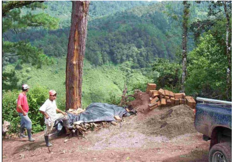
Photo 1: Large quantities of materials are transported to remote sites.
