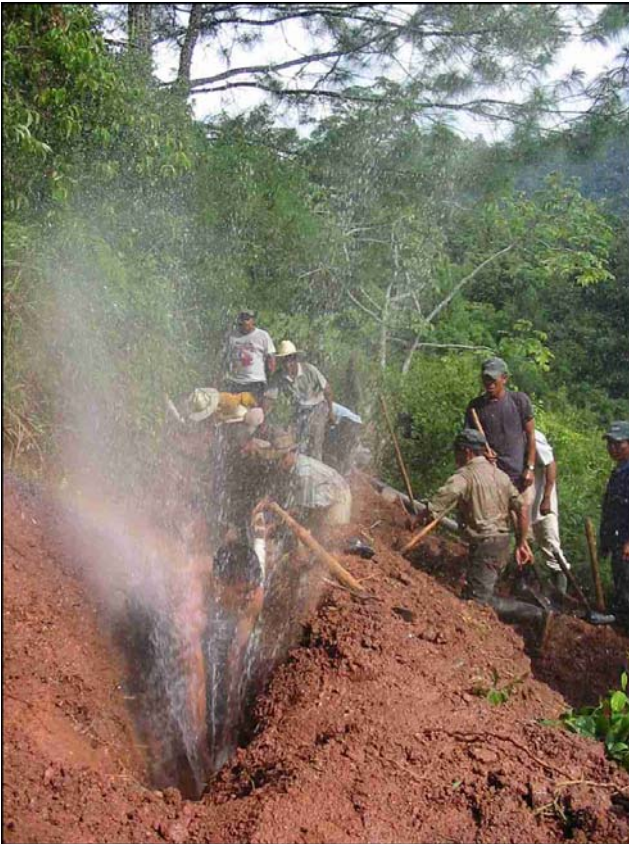
Photo 9: Pipes burst as we try to advance the water to the previous tank site
