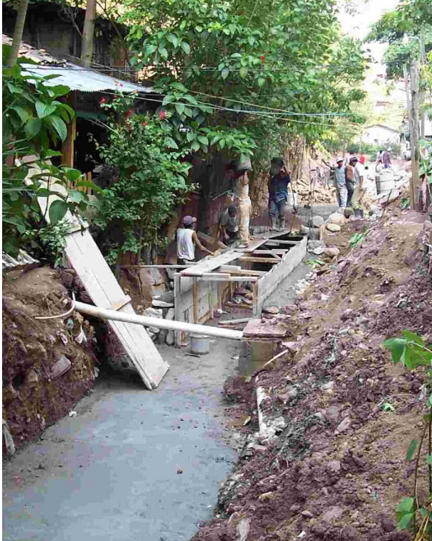
Photo 5: Construction of the storm sewer culvert
