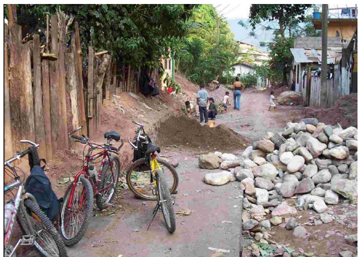
Photo 6: The new culvert turned a opened sewage drain into a path for bike through the community
