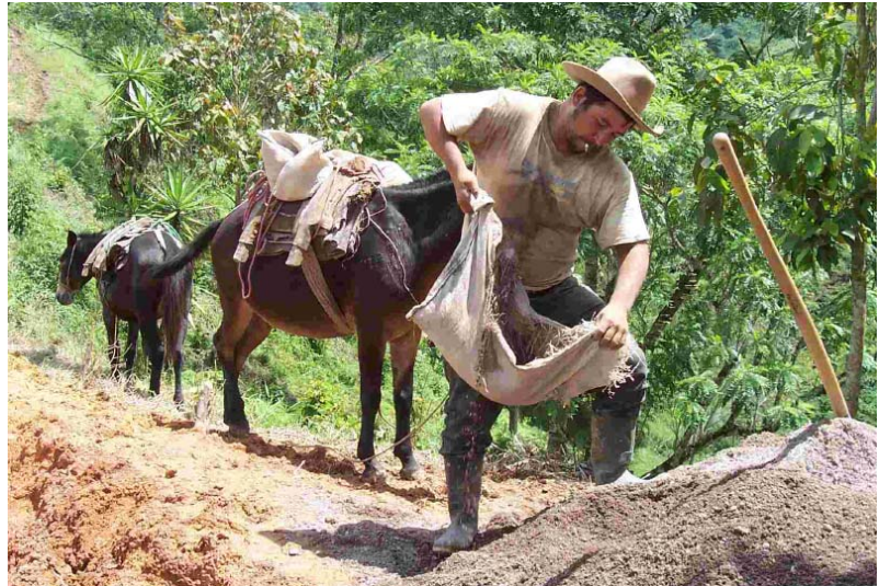
Photo 2: Aggregate is carried by mules and concrete is hand-mixed on site.
