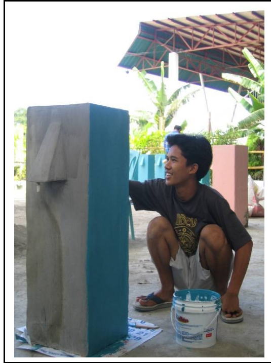
Figure 2: Recently Constructed BSF
