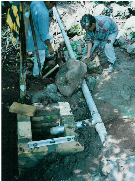
Figure 3.2.5 The construction of a stream crossing of GI pipe, with a clean-out valve on the near side
