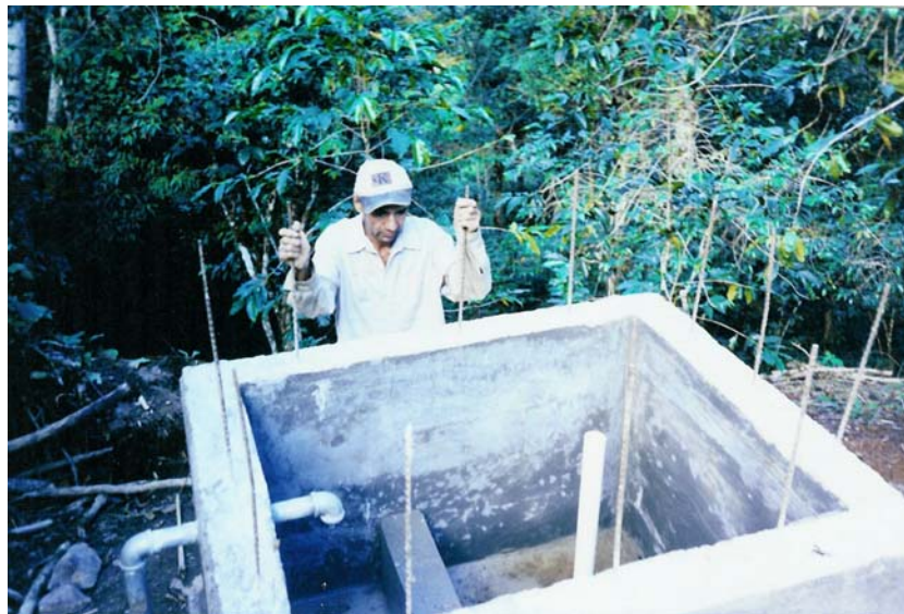
Figure 3.2.6 Construction of a break pressure tank in Honduras
