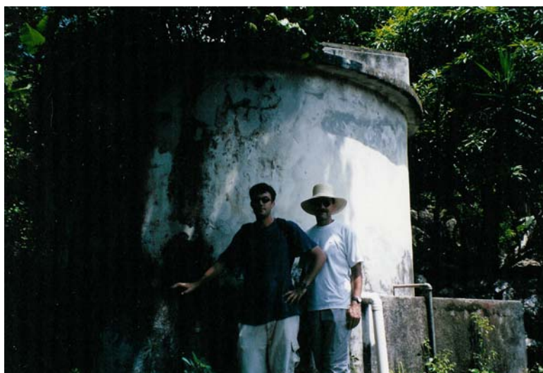
Figure 3.2.7 10,000 gallon storage tank built in Honduras
