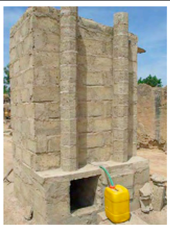
Figure 1.1: Urine diversion for a compost toilet (Photo by Karin Ahlgren, used with permission) (Kvarnstrom et al, 2006: 7)
