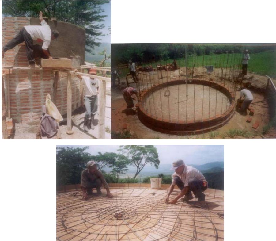
Figure 3-5: Construction techniques of tank walls and roof for 10,000 gallon tank to serve 150 houses. Upper left photo shows mortar being applied to brick walls, upper right photo shows steel reinforcement in wall, and bottom photo shows steel reinforcement for concrete roof.
