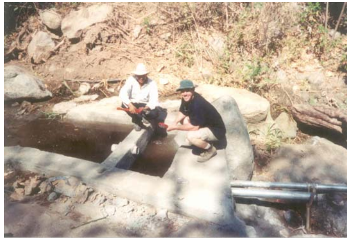
Figure 3-3: Example of concrete surface-water source with settling chamber for community of 150 houses, feeding a tank of 10,000 gallons, with capacity of tubing to carry 50 gallons per minute. Approximate flow rate of source as shown = 75 gallons per minute.
