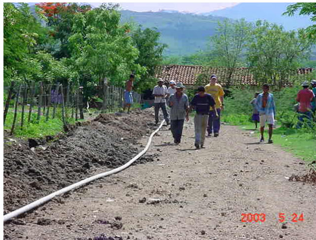
Figure 3-6: 2” PVC tubing ready to be placed in 3’ deep trench for distribution line in a community of 50 houses.
