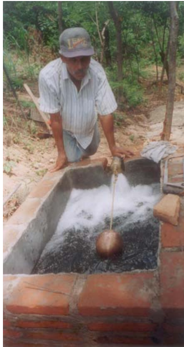
Figure 4-8: Pressure-break tank with 2” diameter float valve with valve currently open due to demand by houses downstream from pressure-break tank.
