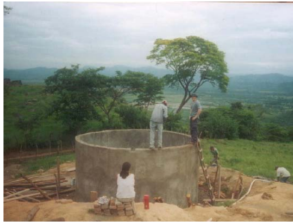
Figure 4-5: Construction of 10,000-gallon tank for community of 150 houses
