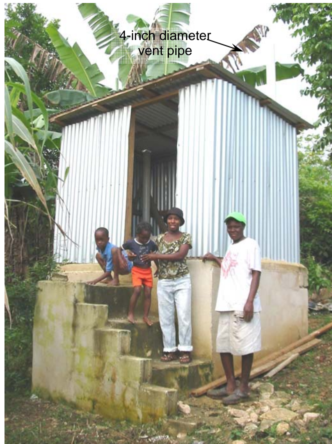
Figure 11: Ventilated Improved Double Pit Latrine (VIDP), Trelawny, Jamaica. Photo courtesy of Ben Liu, 2002.
