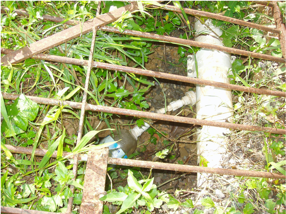
Figure 4-2 Retrieve effluent collection apparatus showing pipe tap and collection bottle under a steel grill. (Photograph by author.)
