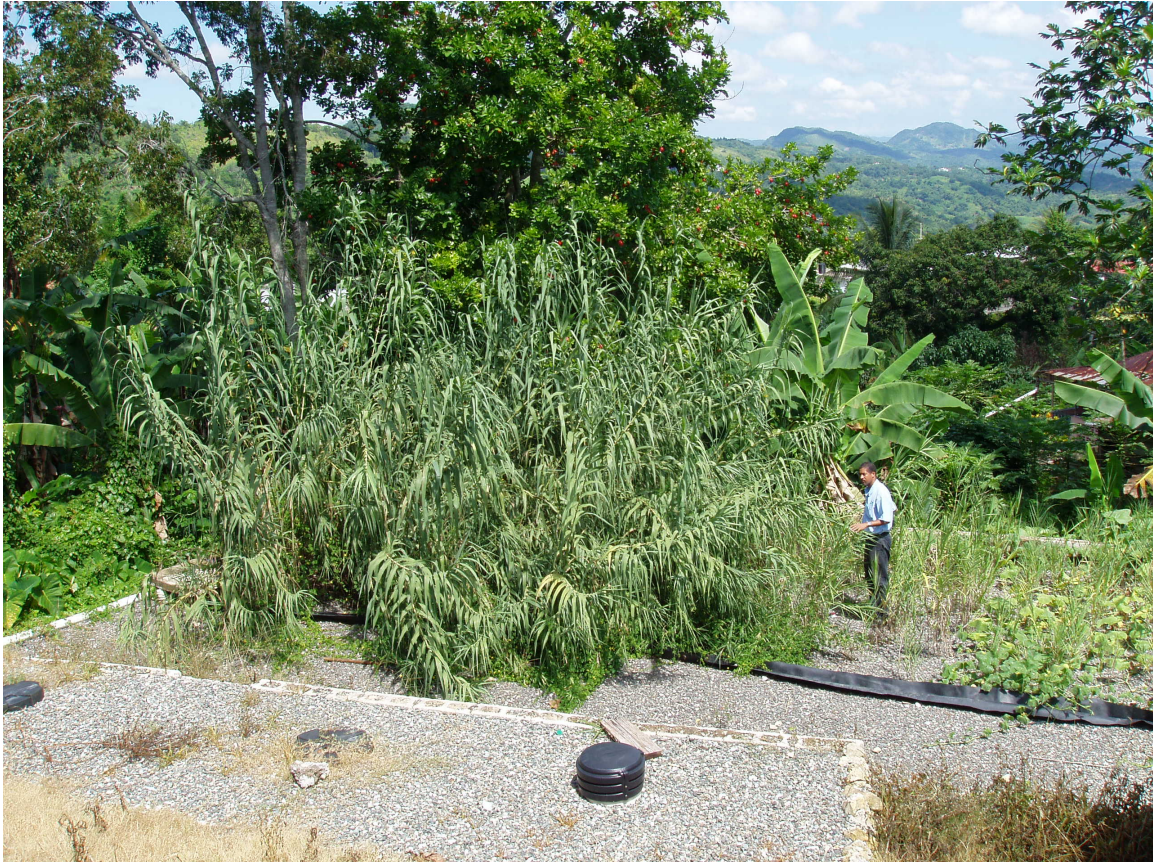
Figure 3-5 Pisgah wetland at the beginning of the evaluation with ten month old wild cane. The design engineer is standing at the mid-wetland sample point used for collecting the “effluent” sample. (Photograph by author.)
