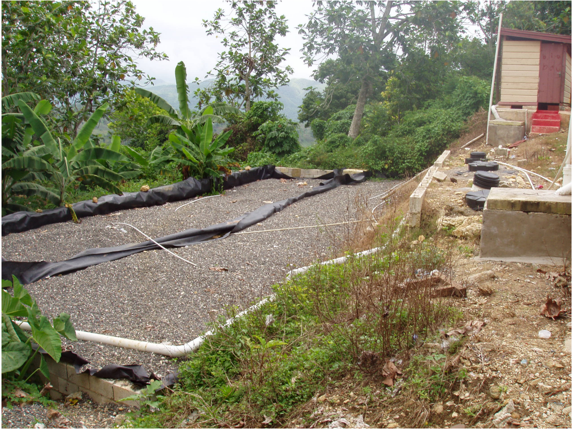
Figure 3-4 Pisgah wetland beds before planting. The black plastic liner running down the middle separates the two beds. (Photograph by author.)
