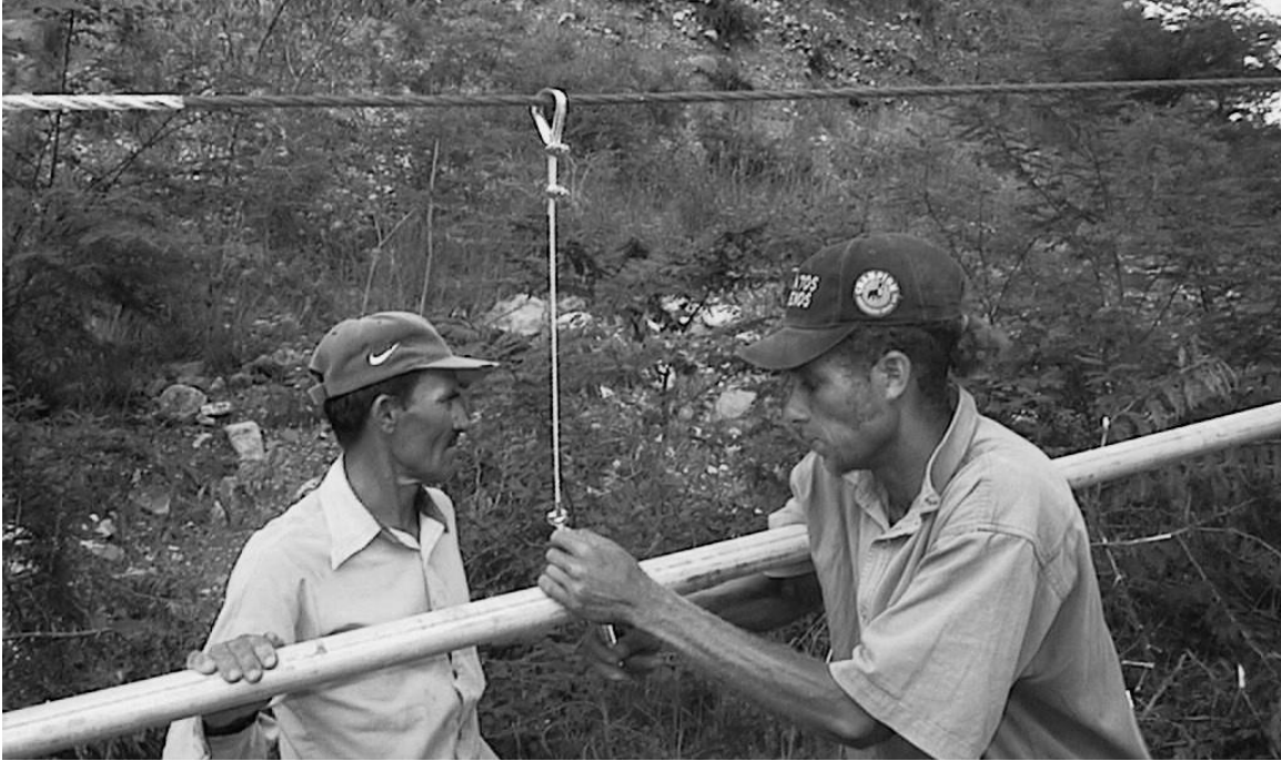
Figure 5-9 Two Dominican construction technicians attach a galvanized pipe to the main cable. (photo by Eric Zalkin)
