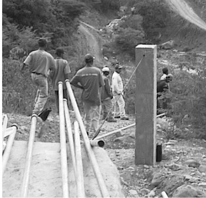
Figure 4-12 A square concrete column and anchor with cable attached. (photo provided by Eric Zalkin)
