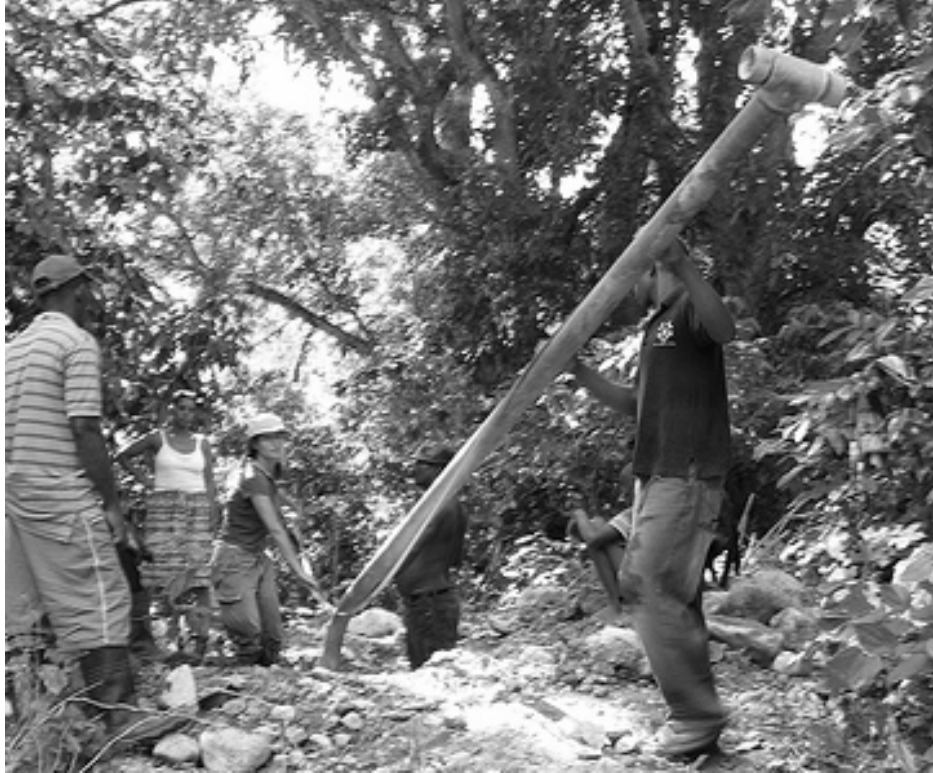
Figure 3-5 Christina Osborn measures the salvageable section of a tree-damaged column. (photo by Kristina Katich)
