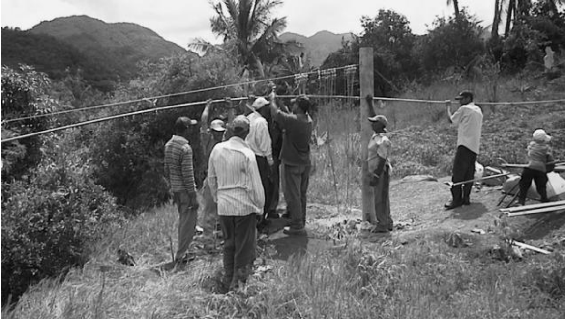
Figure 5-10 Pipes are connected while a crew waits to push out the next length. (photo by Eric Zalkin)
