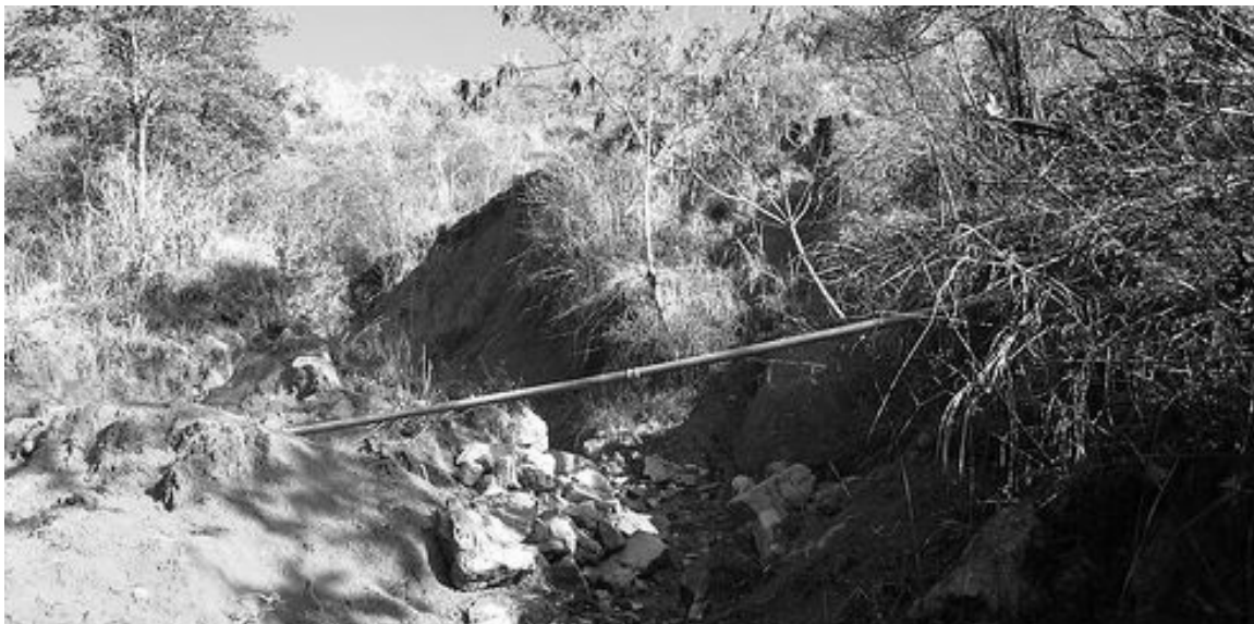
Figure 1-3 A double cantilever crossing over a rockslide. (Photo provided by Kristina Katich)
