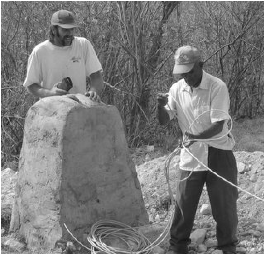
Figure 3-4 The wrong way to unroll a cable. (photo provided by Kristina Katich)
