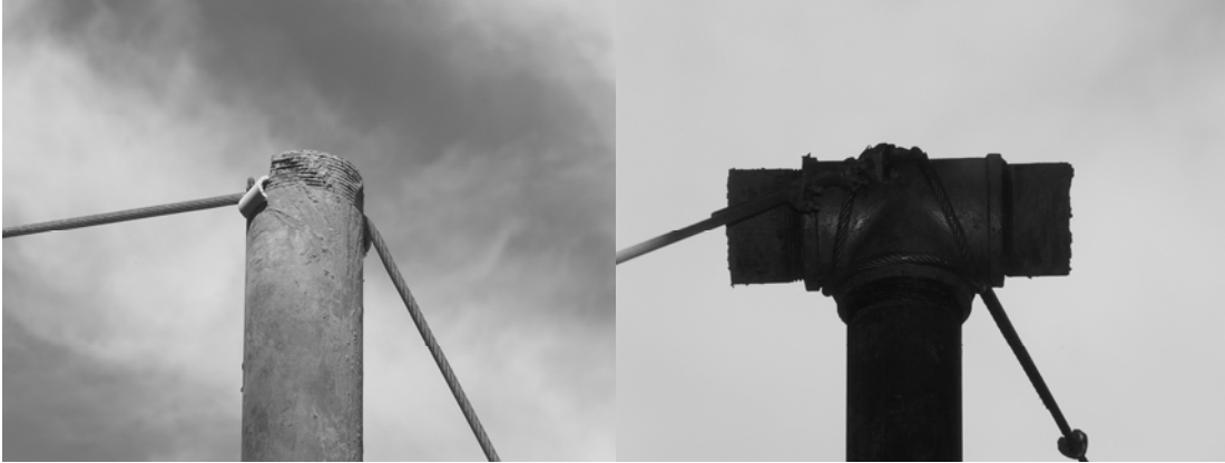
Figure 4-10 Two options for attaching cable to the top of a steel column.
