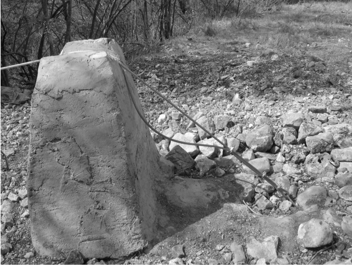
Figure 4-19: A tower and slab type anchor mass constructed of native limestone rubble and covered with a coat of cement plaster.
