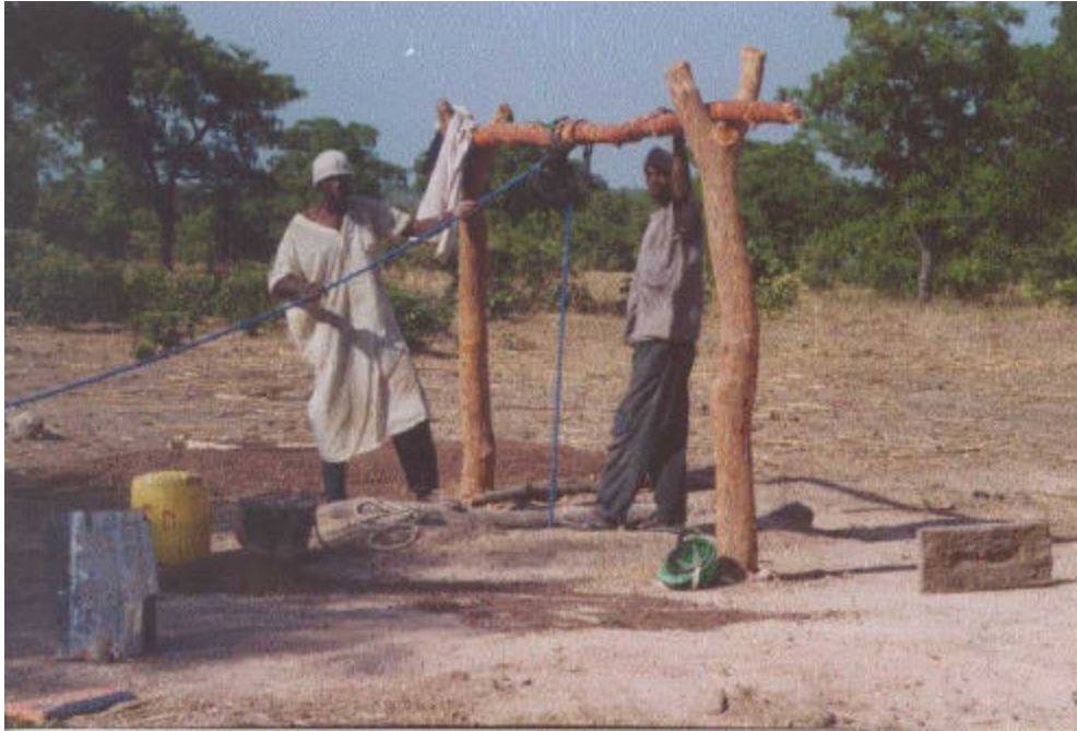
Figure 3.1: Well Repair Project
