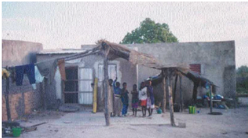
Figure 4.6: House with Corrugated Metal Roof
