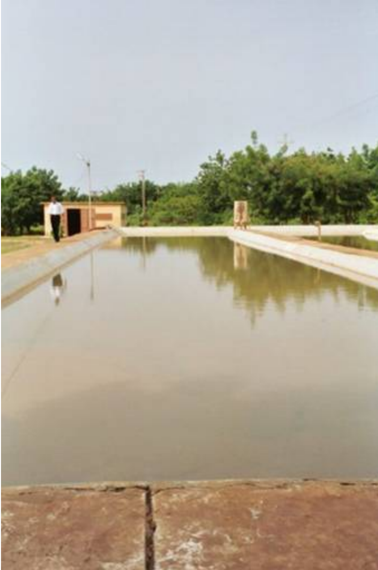
Figure 3-3. Sedimentation Basin at the Kayes Water Treatment Plant
