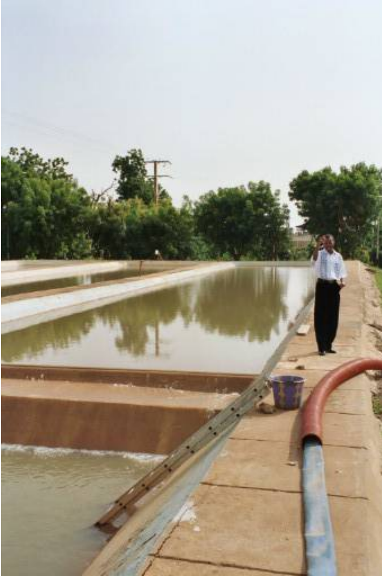
Figure 3-4. Sedimentation Basins at the Kayes Water Treatment Plant under Mr. Diarra's supervision.
