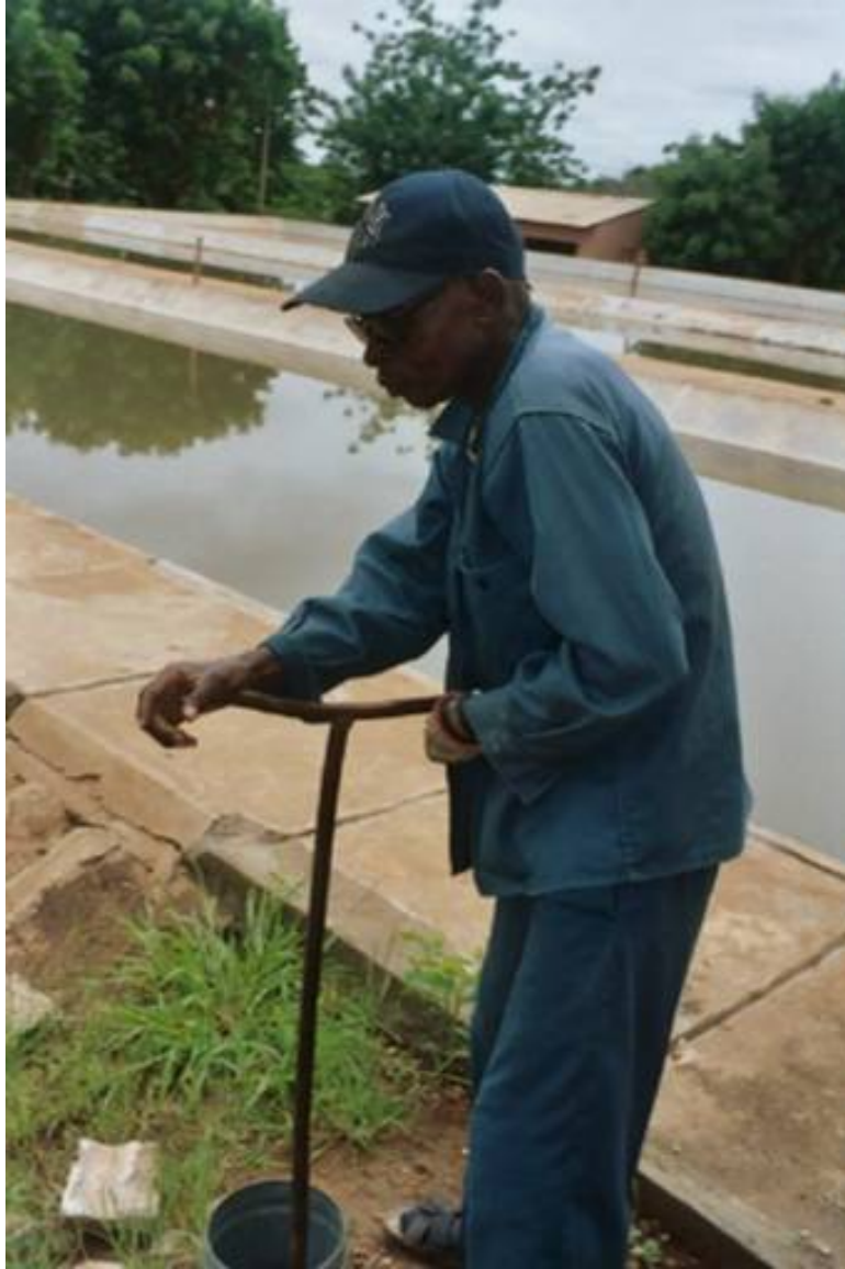
Figure 3-2. Photo of Solid Residuals Management at the Kayes Water Treatment Plant which shows Seydou Diawarra turning the valve to release the solid residuals to the outlet to the Senegal River.
