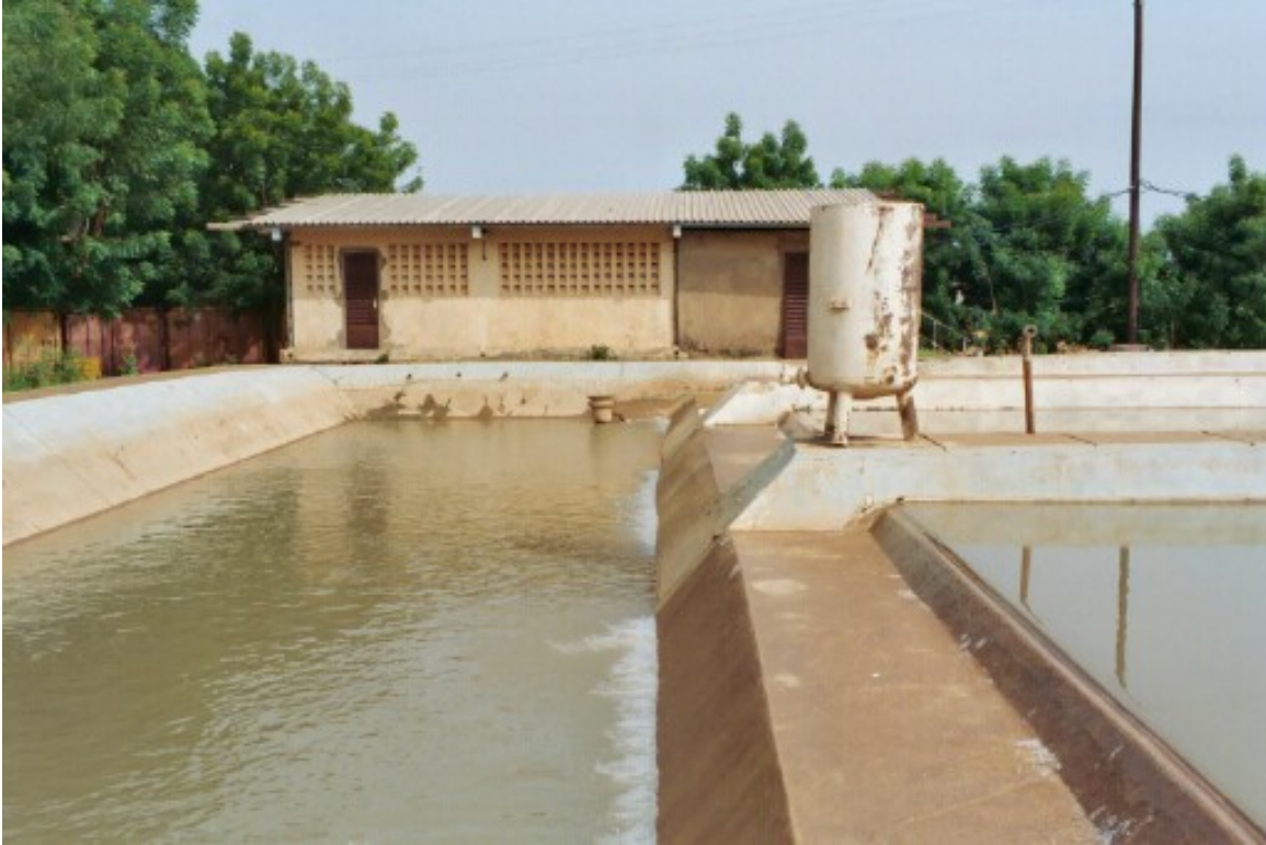
Figure 3-5. Base Sedimentation Basin at the Kayes Water Treatment Plant
