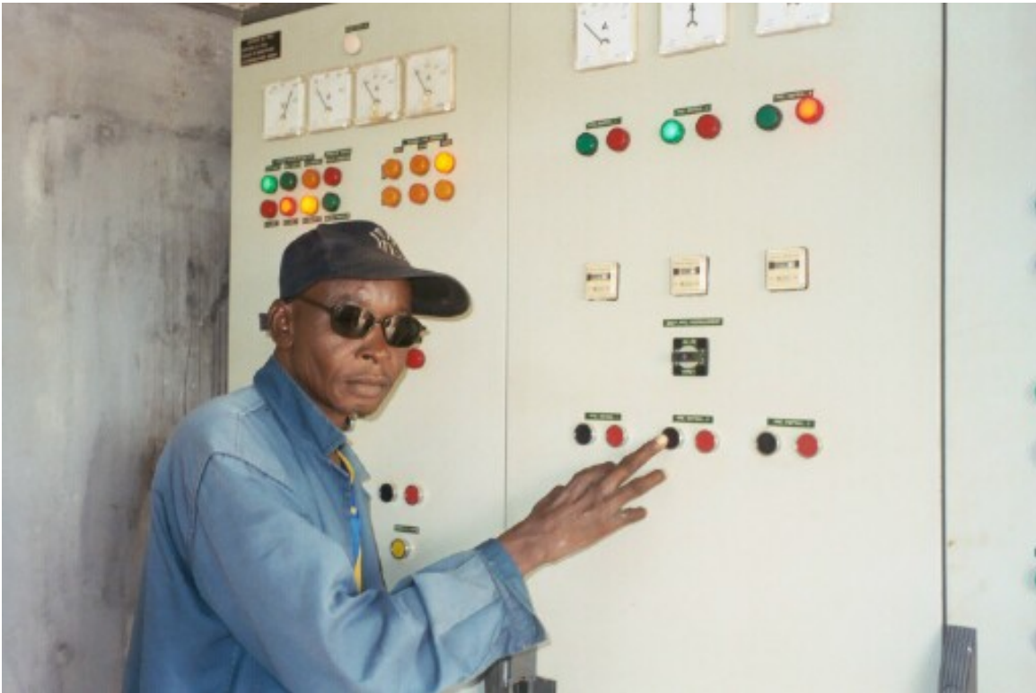
Figure 3-11. Treatment Plant Technician, Seydou Diawarra, at the flow controls of the Water Treatment Plant.
