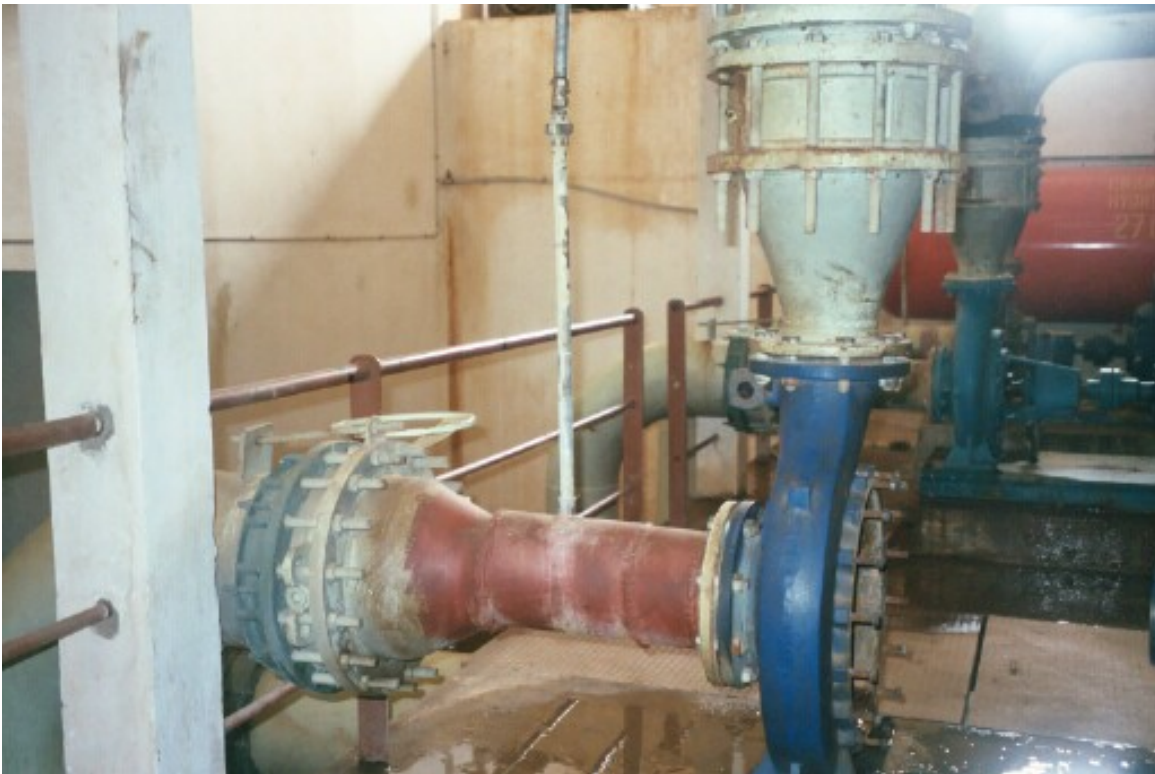
Figure 3-9. Main pumps to the Kayes' Distribution System
