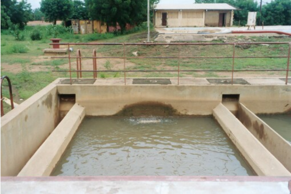
Figure 3-6. Sand Filters at the Kayes Water Treatment Plant
