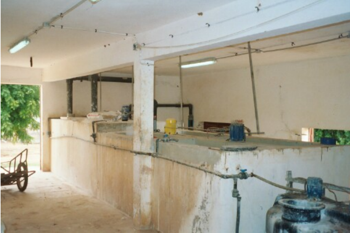
Figure 3-8. Chlorine Mixing Basins at the Kayes Water Treatment Plant
