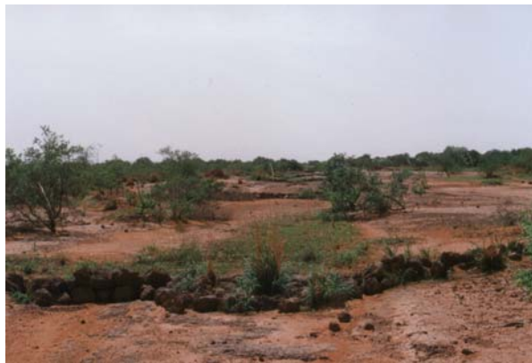
Figure 20: Construction of Stone Walls in a Gully for Plant Production
