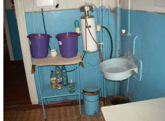
Water heater for sink
