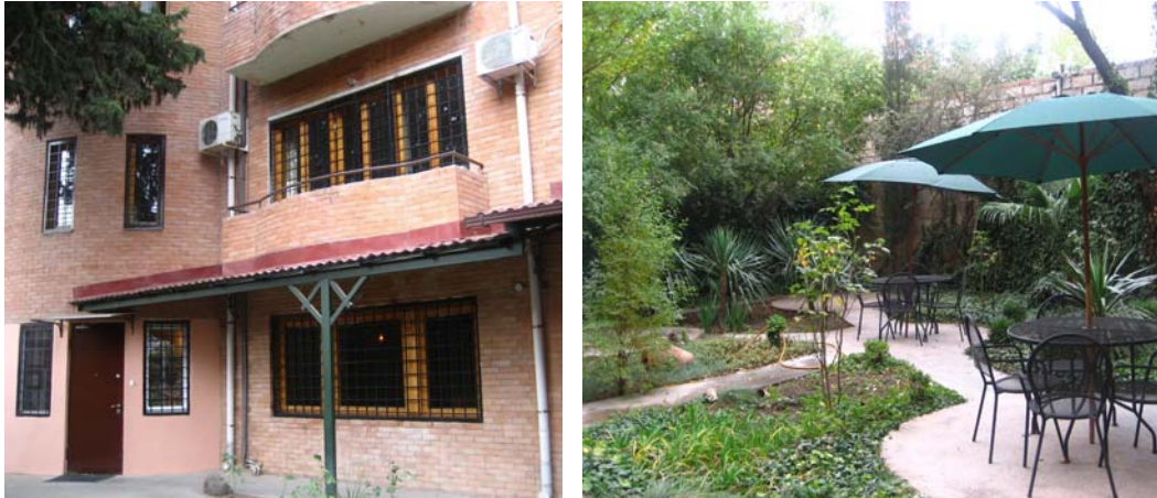
Peace Corps/Georgia office building (left) and garden (right)
