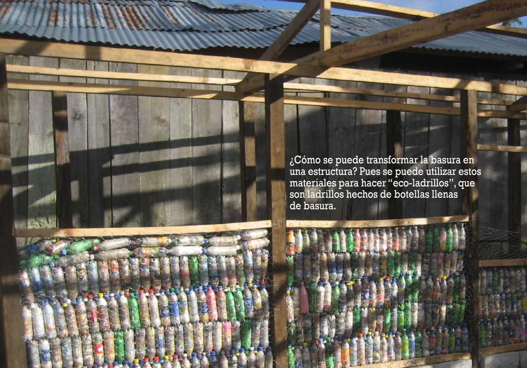
The image shows a wooden frame structure under construction. The walls are made of plastic bottles, which are used as 'eco-bricks'. The bottles are arranged in a grid pattern, with some bottles being clear and others colored (green, blue, red). The structure is built on a wooden frame with a corrugated metal roof. The background is a dark wooden wall. The text is overlaid on the right side of the image.
