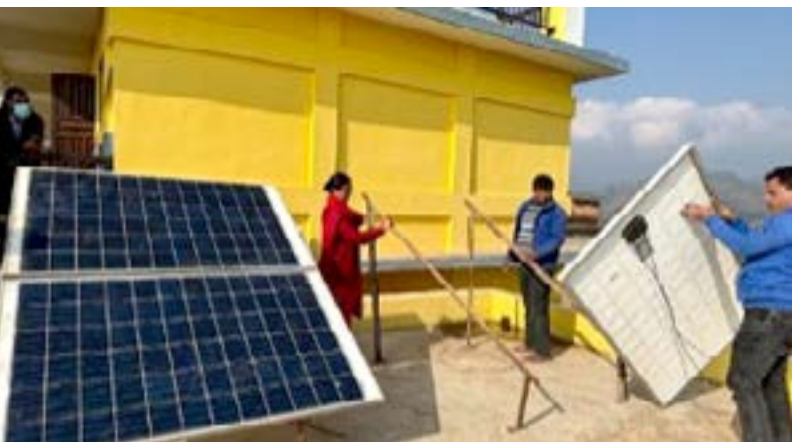
Installation of solar panels to help power the school's new technology.
