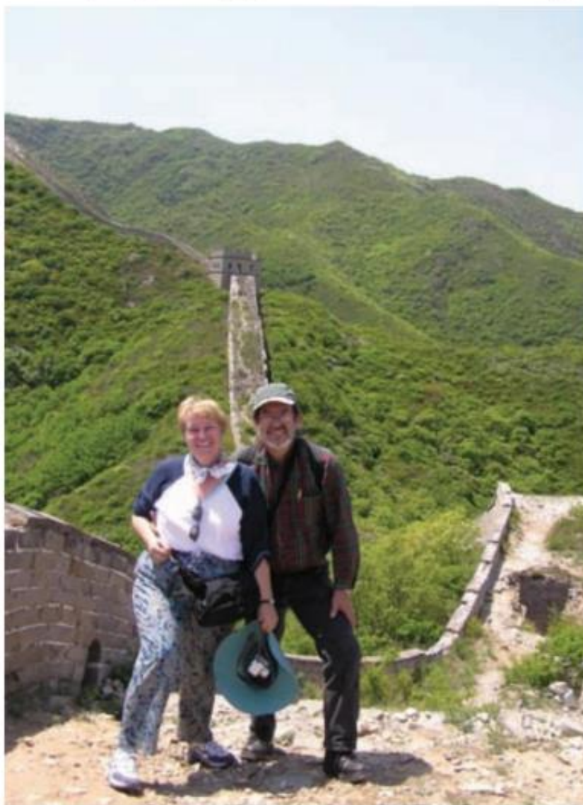
Evelyn and Walter at an unrepaired wall along the Great Wall of China.
