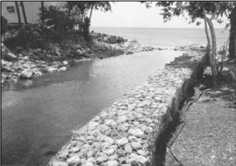
Gabion to reinforce stream bank
