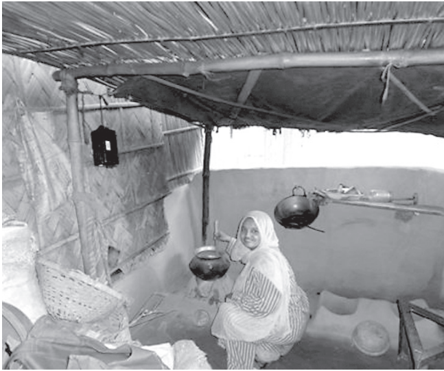
Figure 10: Example of good ventilation with gap between kitchen wall and roof, Bangladesh. Photo courtesy of Aprovecho Research Center
