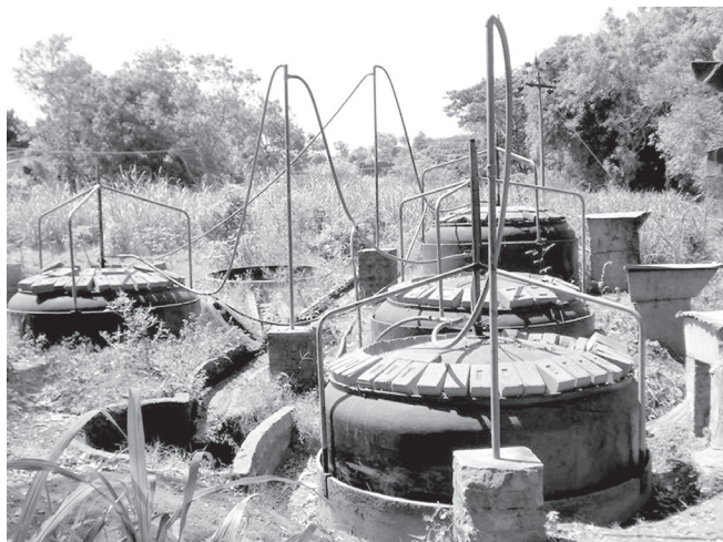
Figure 7: Biogas generation. Photo courtesy of Aprovecho Research Center
