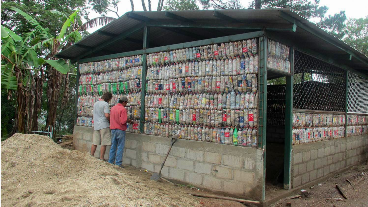
Classroom built partially with eco bricks
