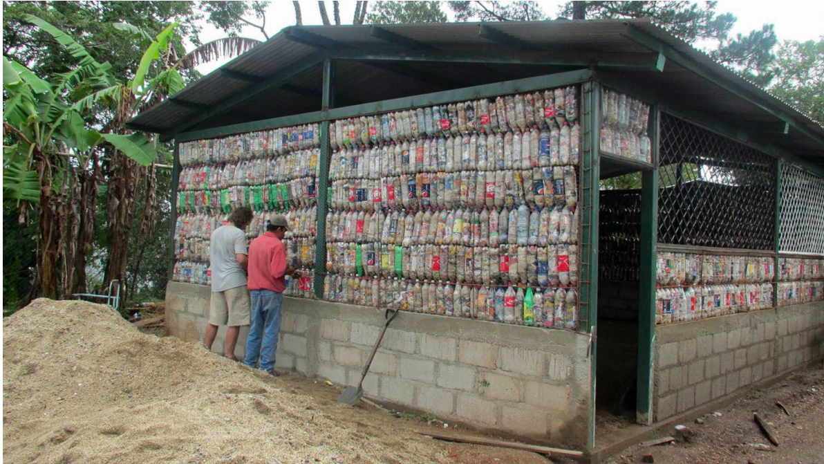
Classroom built partially with eco bricks
