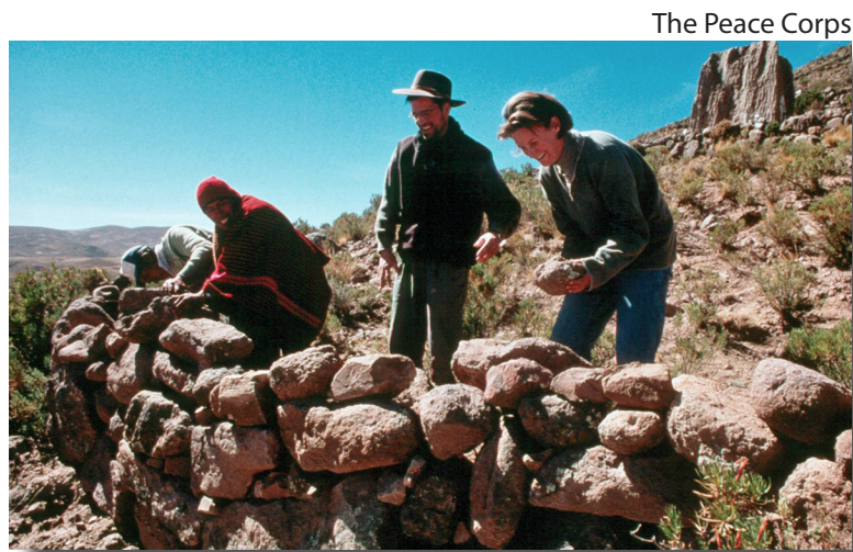
Figure 4-9. A Loose Rock Wall Barrier
