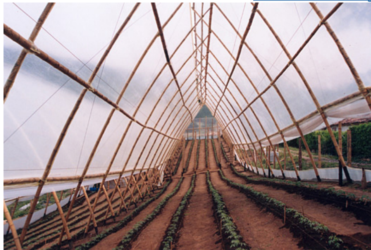
Figure 5-4. Construction with poles (instead of finished lumber) is common in tropical countries, especially in rural areas.
