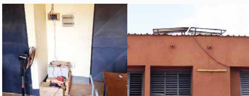
Solar batteries and wiring, and solar panels
