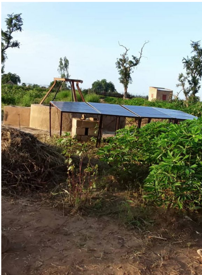
Solar panels installed in the field to power a solar water pump
