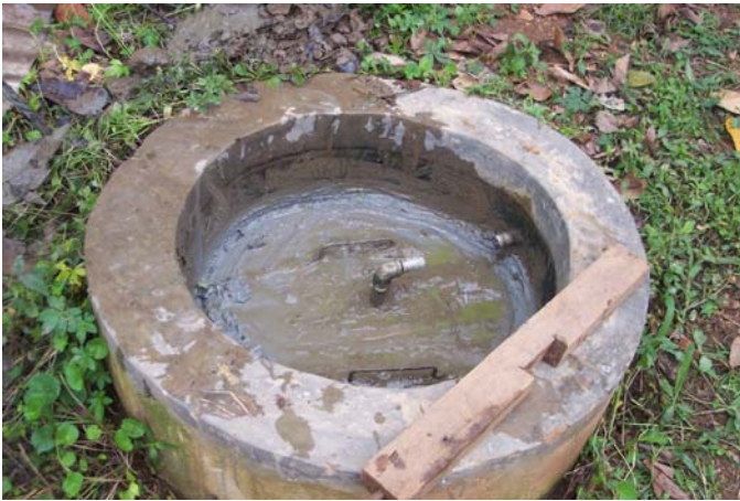
Figure 12: Manhole Cover with Gas Outlet
