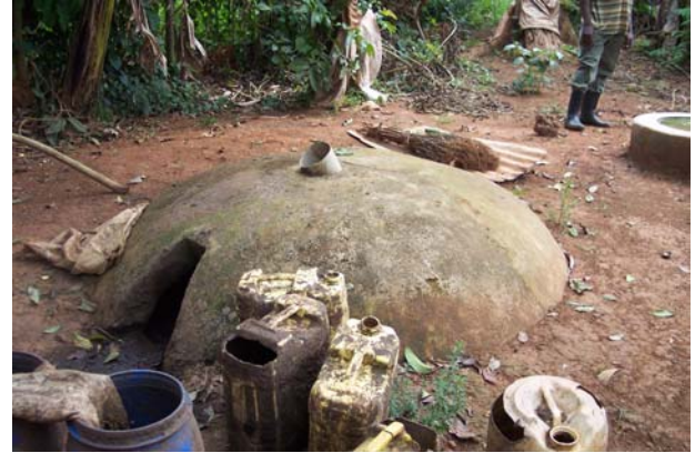
Figure 20: Expansion chamber with jerry cans to transport slurry to field
