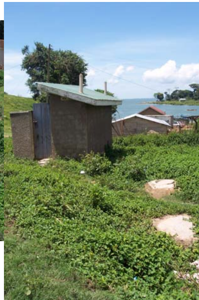
Figure 15: View of expansion chamber, top of digester and latrine house at Katosi
