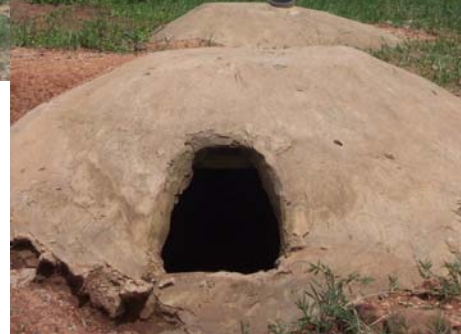
Figure 9: Opening for expansion chamber at Jim's Education Center
