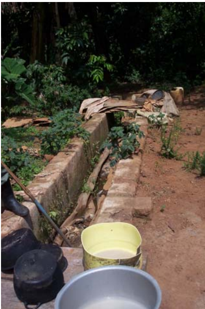
Figure 17: Trench for tubular system for James Mugerwa
