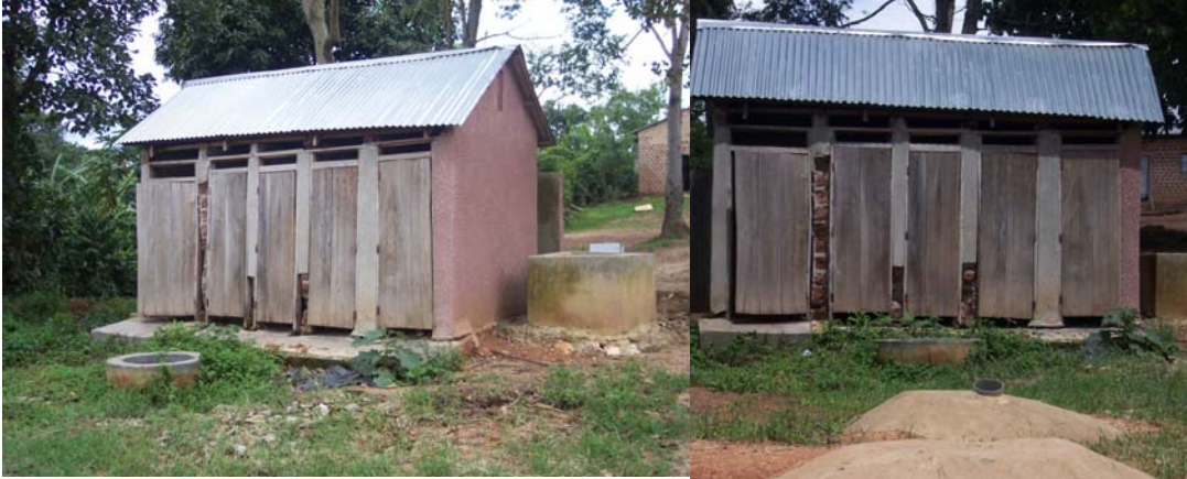
Figure 8: Latrine house at Jim's Education Center
