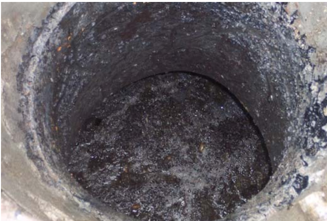
Figure 13: Inside View of Digester
