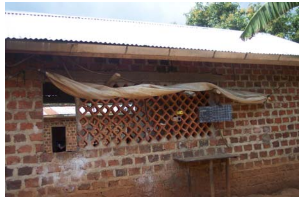
Figure 18: Gas storage for tubular system for James Mugerwa
